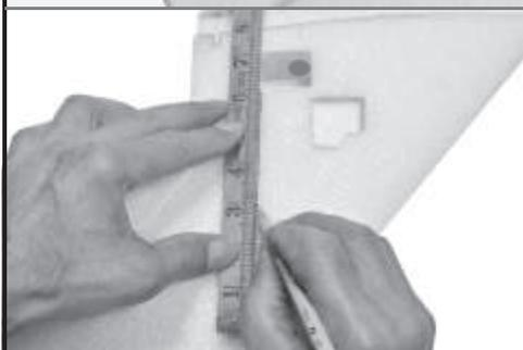
Skip this step if a 72 MHz receiver with a long antenna is being used. The antenna tube is for some 2.4 G radios only. 2.4G receivers with one or two long antenna wires will work with the tube. Locate the red antenna tube in the parts bag. Trim the length to 6". Measure 6" spanwise from the corner of the bay receiver toward the tip. Make a 6" mark along the straight-edge.
