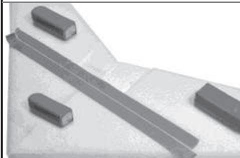
Mask the spar channel on both sides with masking tape.
